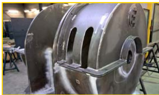
Lassamenstel mantelblok 45t Welding assembly mantle block, 45t
